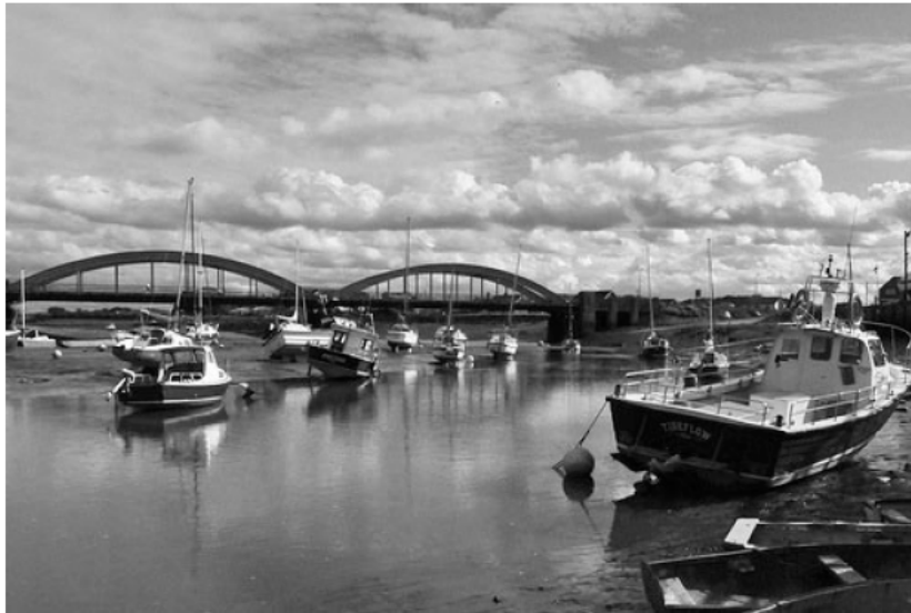
The Foryd Bridge and Harbour with a rising tide. 1
